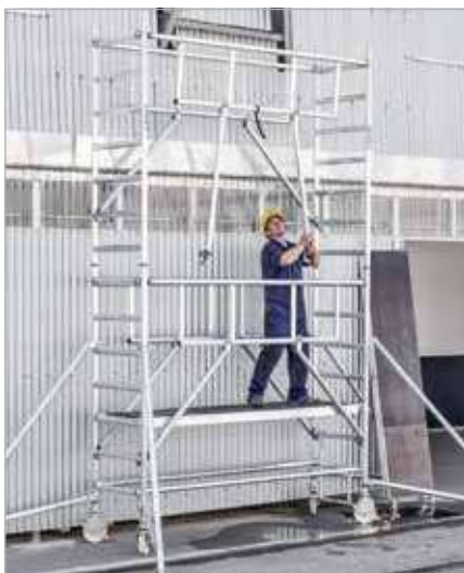
1. Insert advanced guardrail
