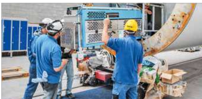
Supervising the tower installer
