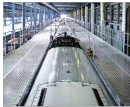
Roof work scaffolding, length approx. 920 m, for ICE maintenance
