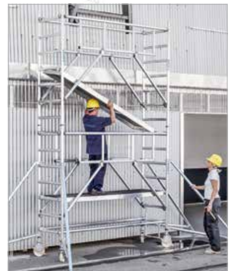
3. Hook in platform from a secured position
