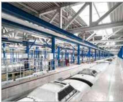
Roof work scaffolding, length approx. 1,300 m for 3 tracks
