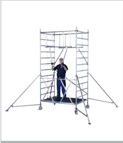
1. Hook the advanced guard rail from the lower platform
