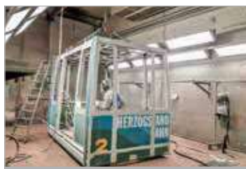
Preparation for applying anti-corrosion protection
